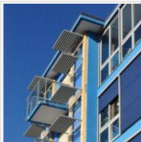
Design and energy retrofitting
